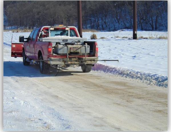
Vehicle travel across snow covered wooden matting, where lime chips have been applied.
