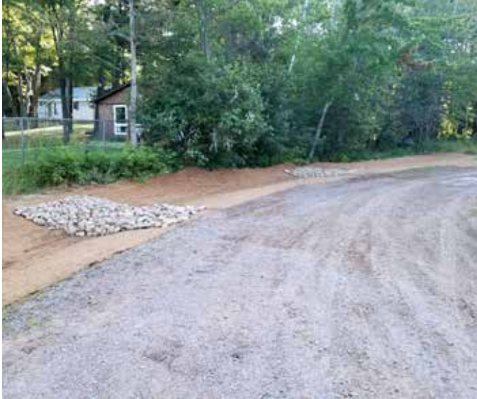
Grassed waterway adjacent to Sand Lake. Photo courtesy of Florence County.
