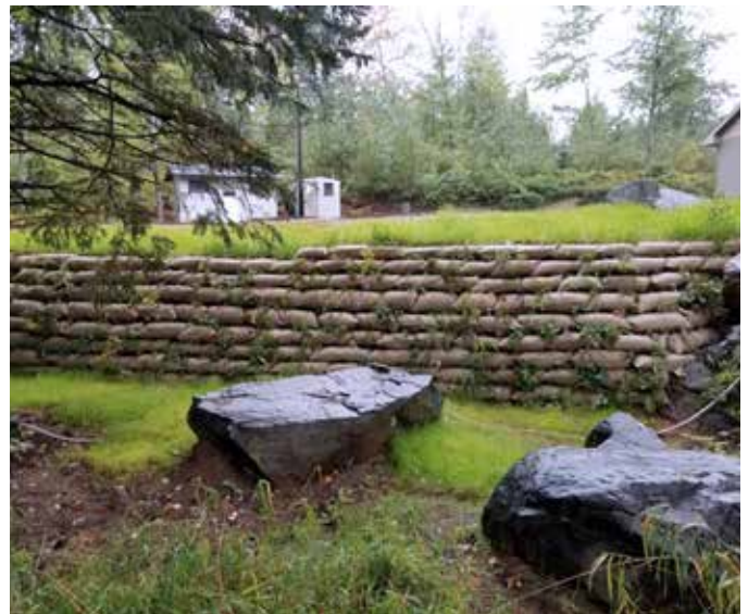
Geotextile wall in Florence County. Photo courtesy of Florence County.
