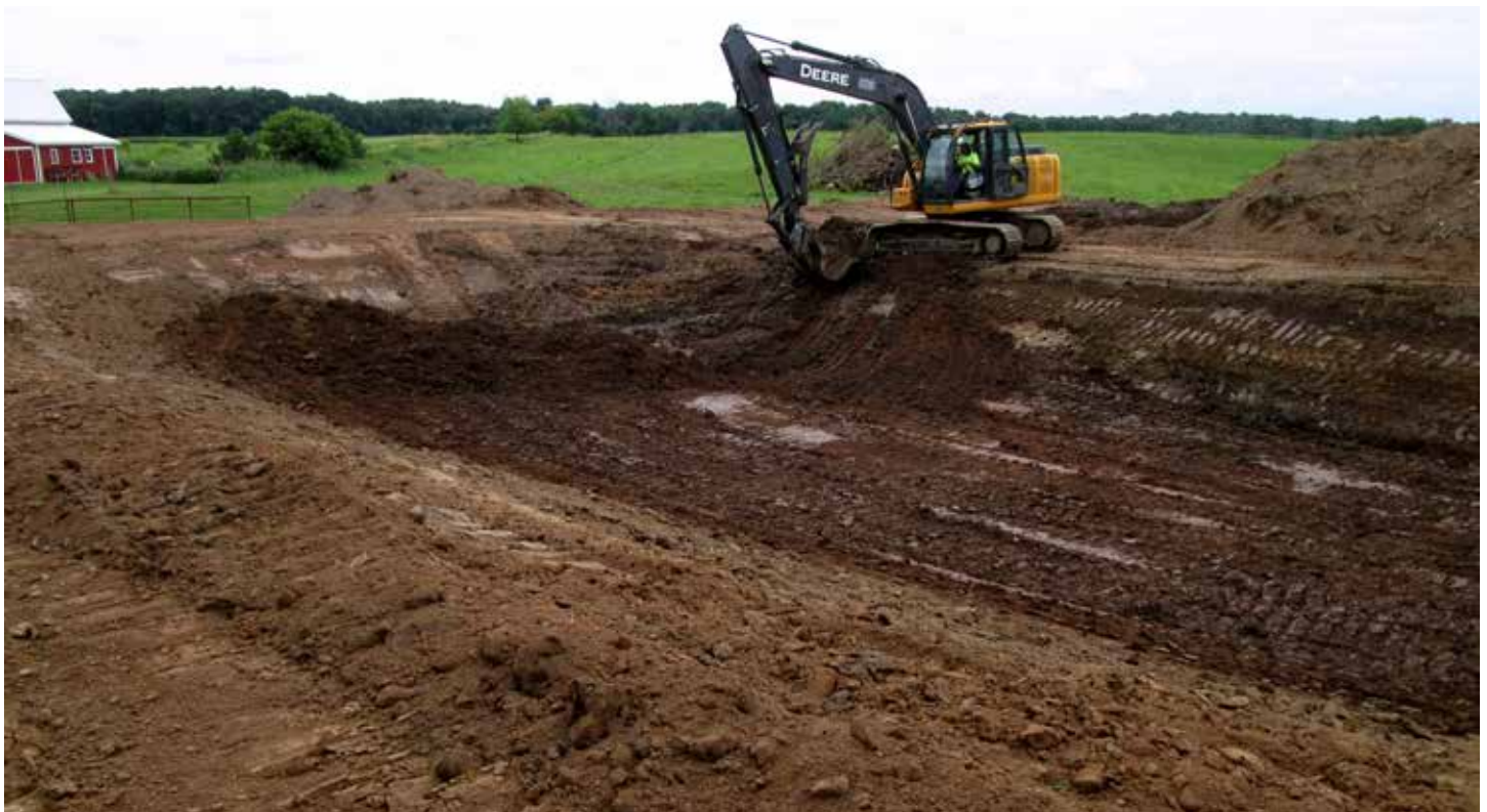
A manure storage abandonment. Photo courtesy of Polk County.
