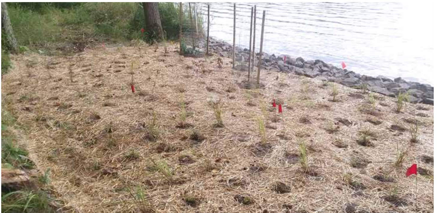
Native planting and streambank stabilization. Photos courtesy of Douglas County.
