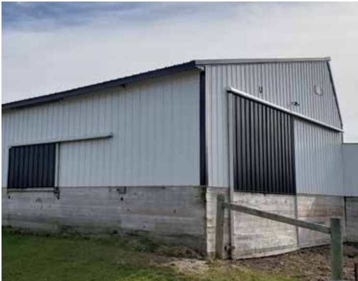
BEFORE - Installing roof gutters at the Laeser property. Photo courtesy of Iowa County
