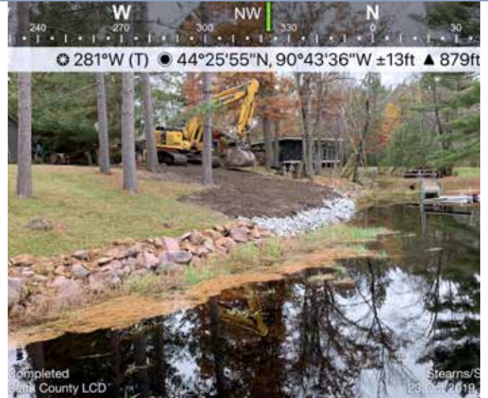
Completed shoreline project on Arnold Creek. Photo courtesy of Clark County.
