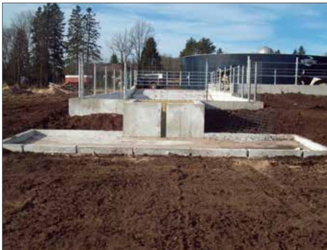
Feedlot spreader box. Photo: Tom Fratt, Ashland County Land and Water Conservation Department
