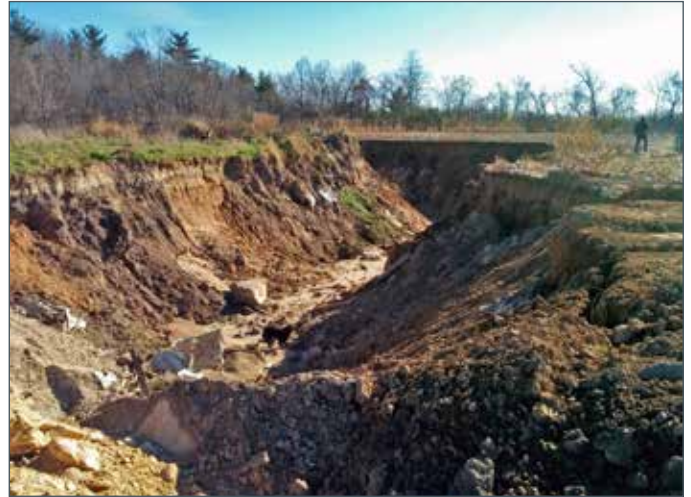
Eroded Channel: 22-foot deep gully cutting through the Swoboda's crop field
