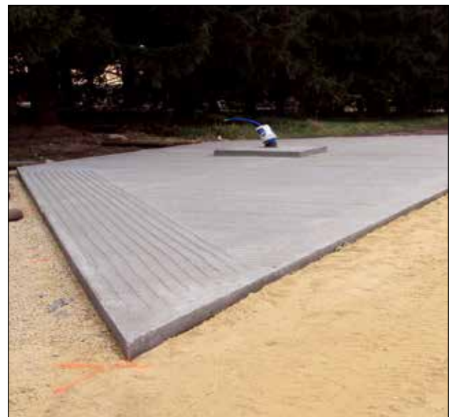
Feed lane with newly installed watering station
