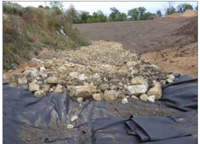
Bottom of the channel, during placement of geotextile fabric and riprap
