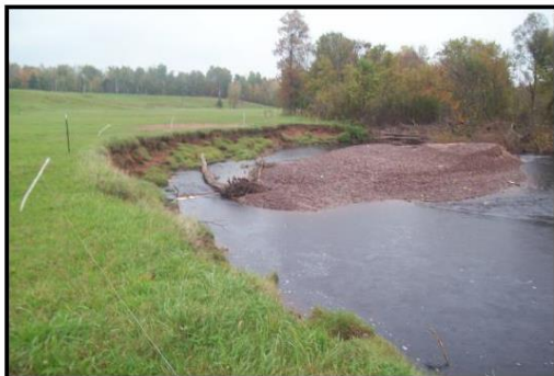
Above right: Root Wads laid on streambed and duckbills anchored into the bank.
