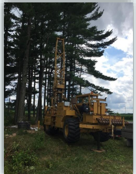
Above: Drill rig with operator installing a new well.
