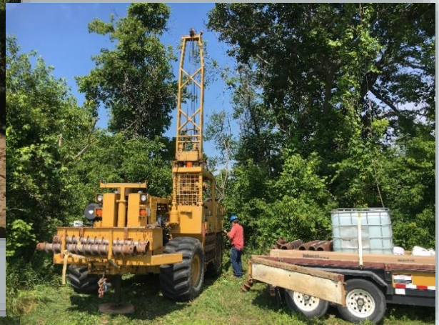
Above: Drill rig with operator installing a new well.
