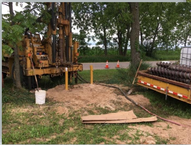
Above: Drill rig and two newly installed monitoring wells.
