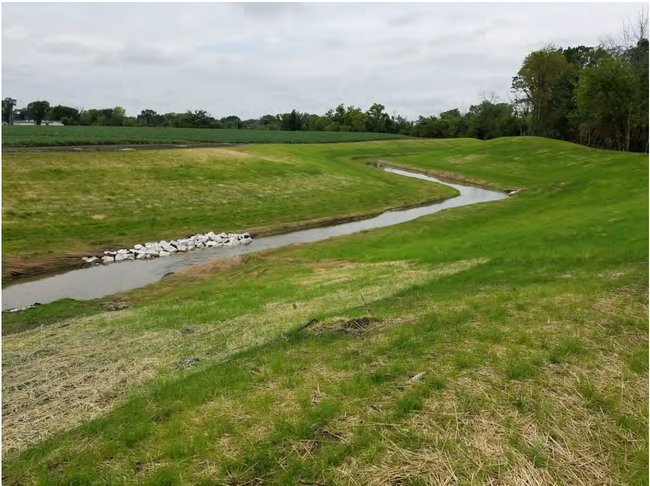
Oakcrest Creek Restoration – Remove legacy sediment, grade/seed eroding banks, create two-stage channel
