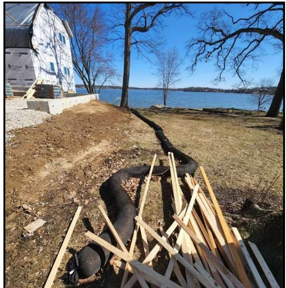
INCORRECTLY INSTALLED SILT FENCE.
