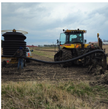
Tile installation for waterway
