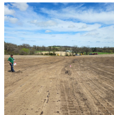
Photos: Sara Wilhelm Tony Pillow inspecting waterway grading
