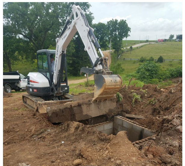
Photo: A non-compliant well pit being decommissioned after the water well was sealed with bentonite
