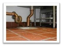
Air gaps installed in wastewater lines of food preparation sinks, dipper wells, ice bins and warewash machines.
