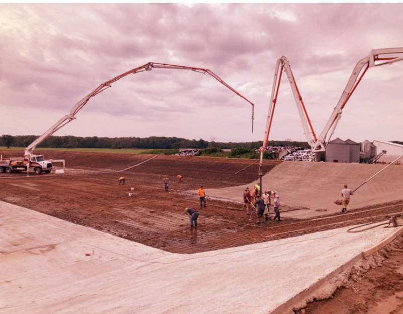
Concrete liner being poured.
