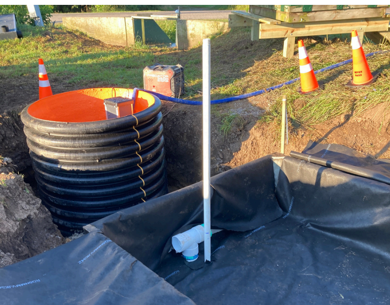
The phosphorus removal system being installed.
