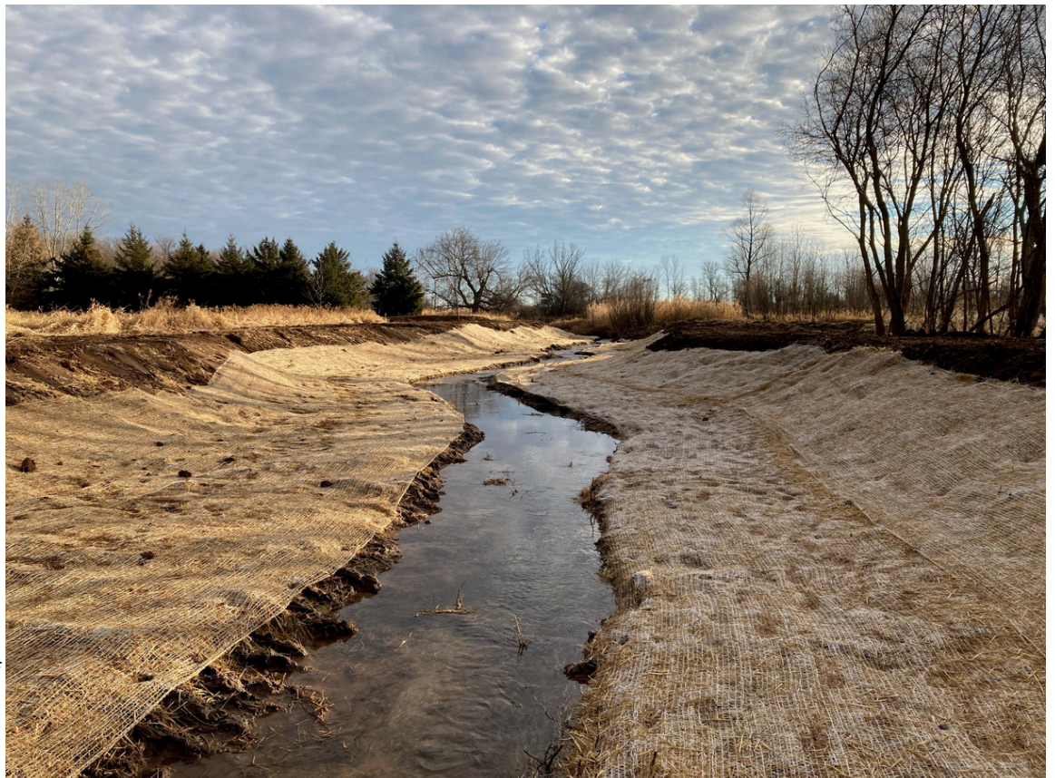
Close up of completed two-stage ditch in Outagamie County.
