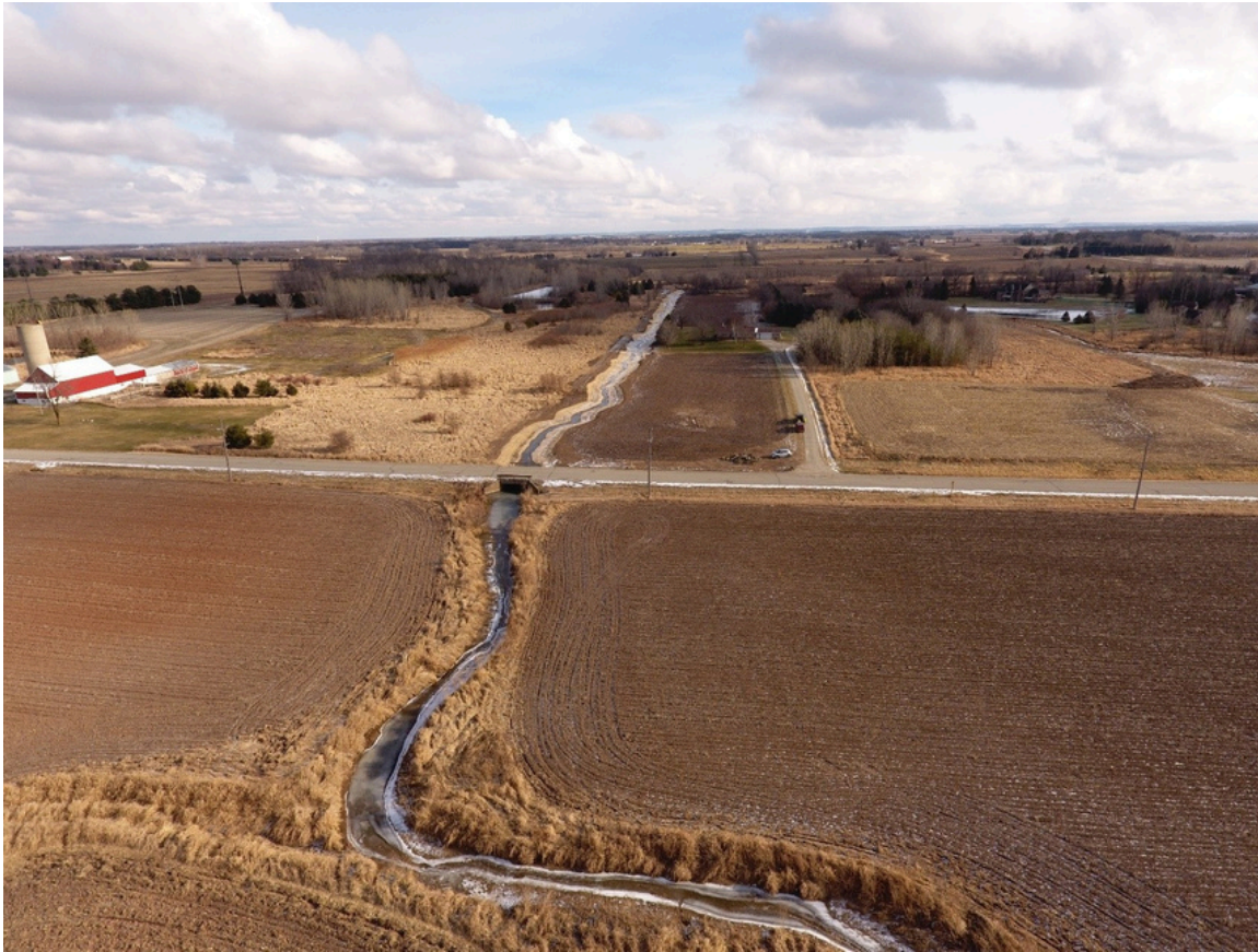
The newly constructed two-stage ditch on top and a conventional dredging on bottom.
