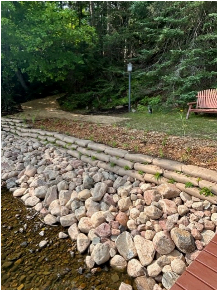
Protected shoreline using riprap and geotextile bags on Butternut Lake. Photo courtesy of Forest County.
