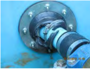
Figure 17. Image of sump boot.
