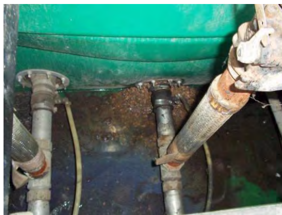
Figure 24. Compromised sump indicating the sump is not “water tight.”
