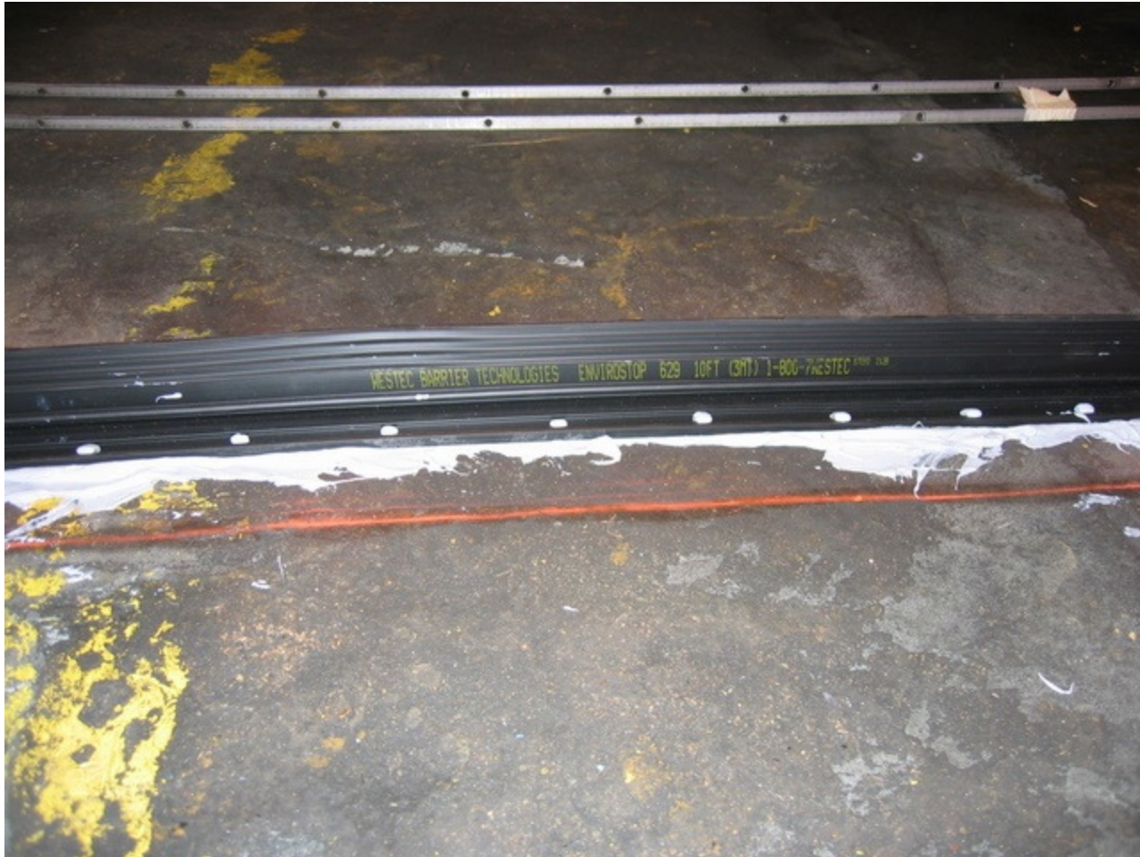
Good Installation – Epoxy Squeezes from behind waterstop
