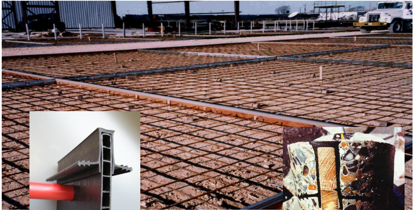
Expansion Board Cap Seal System
