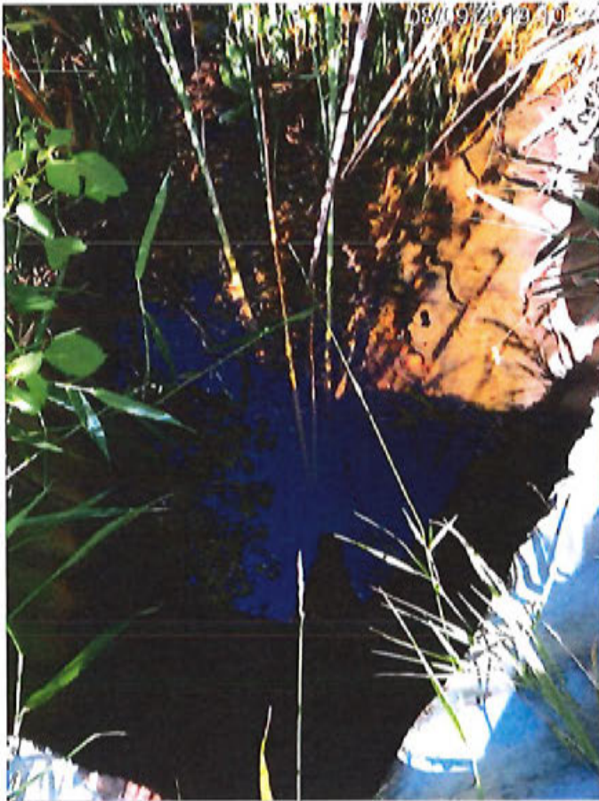
Photo 6 (left). Closeup of water in road culvert on west side of Chestnut Drive north of N7574 Chestnut Drive.
