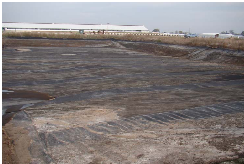
Figure 3.1 Permeable Cover on Lagoon #2, Kewaunee County Farm
