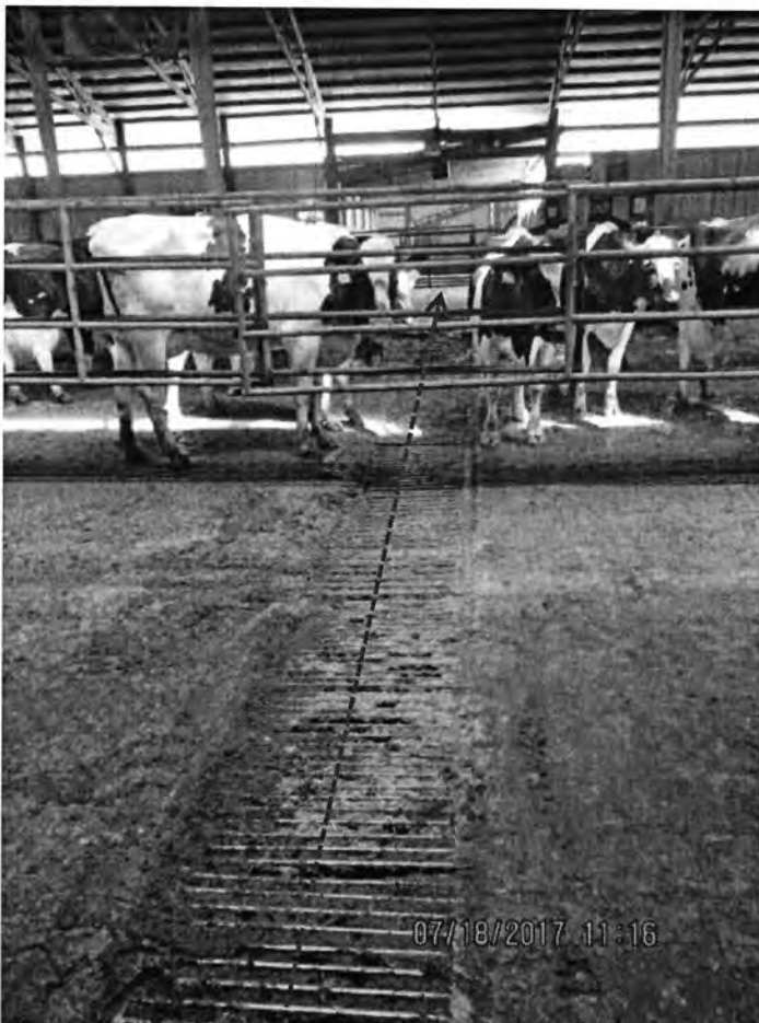
Photo 37: View of the waste collection/manure transfer system inside the freestall barn that discharges directly into outfall/WSF 001. Red dashed arrow indicates the flow direction of waste. Photo direction is north.
