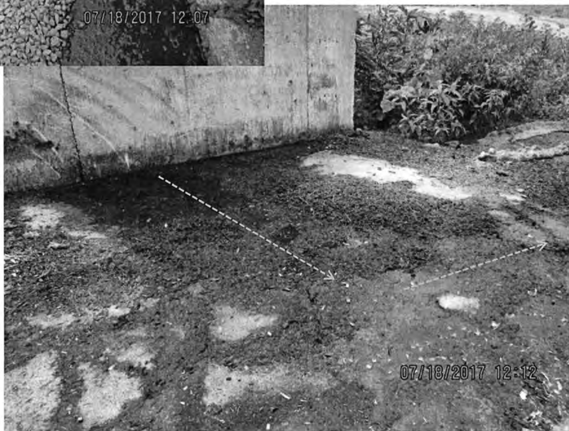
Photo 78: View of the north concrete wall of the feed storage area at the heifer site. Leachate was observed discharging from the wall. Orange dashed arrows indicate flow path of leachate discharge. Photo direction is SW and down.
