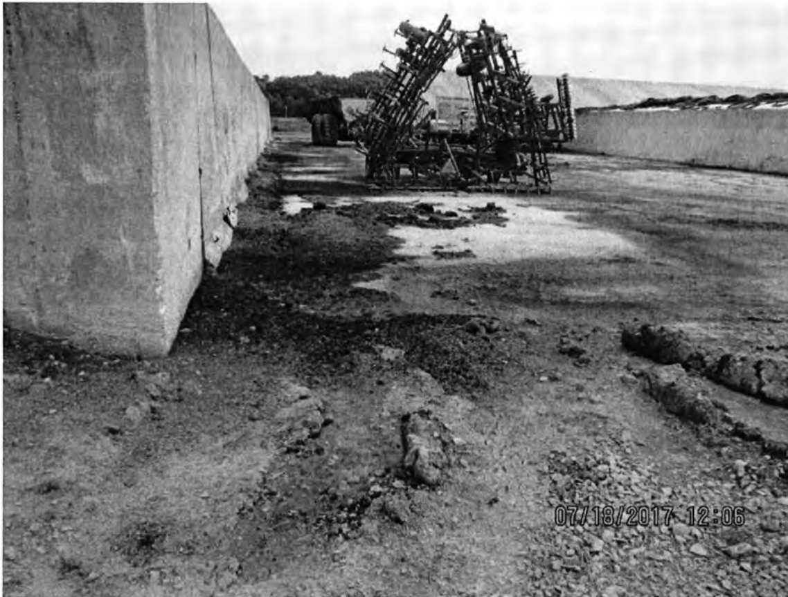
Photo 75: View of a concrete wall from the middle of the feed storage area at the heifer site. Leachate was observed discharging from the wall (black liquid/substance). Photo direction is east.
