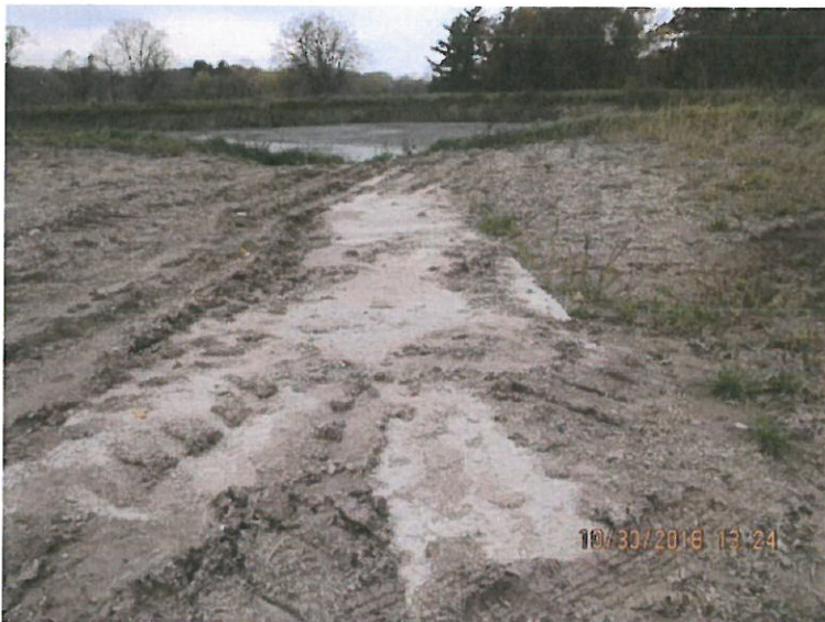
Photo 47: Alternate view of the concrete overflow weir constructed in the waste storage facility to meet secondary containment requirements. Photo direction is west.
