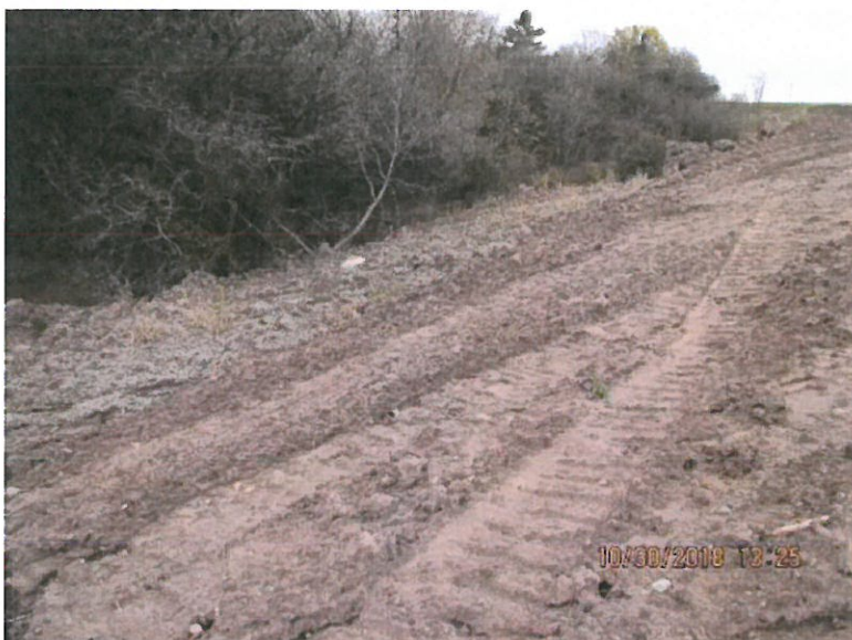
Photo 50: View of a disturbed area east of the waste storage facility that does not contain storm water erosion controls or vegetative stabilization. Photo direction is down and east.
