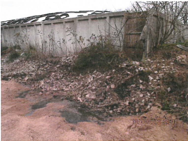
Photo 62: View of the NE corner of the FSA where leachate has been observed discharging during previous site inspections. Leachate is visible ponded on the ground outside the dirt/stone/sand pile outside the wall. Photo direction is west.
