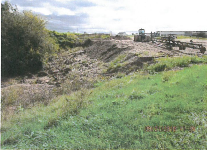
Photo 1: View of a disturbed area without storm water erosion controls vegetative stabilization east of the waste storage facility. Photo direction is east.
