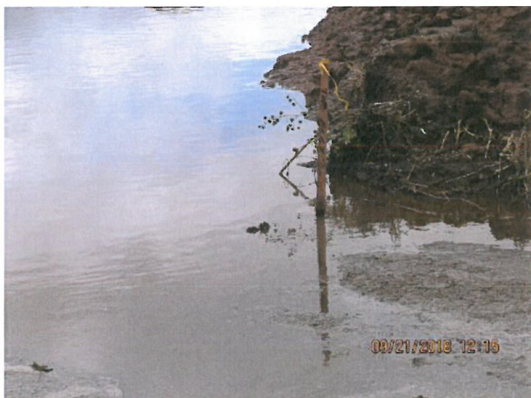
Photo 29: Close up view of a wooden stake in the leachate/process wastewater collection basin that appeared to be a level /volume indicator. Photo direction is SW and down.
