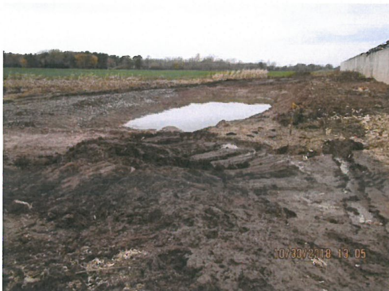
Photo 43: Closer view of the leachate/process wastewater collection basin south of the FSA, showing the regraded inlet area. Photo direction is SW.
