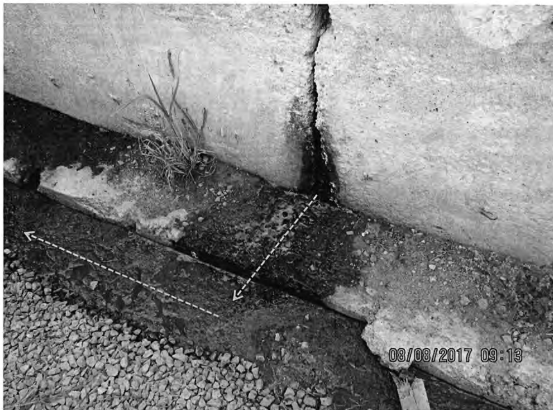
Photo 1: View of a discharge point of leachate / process wastewater on the outer west wall of the feed storage bunker at the heifer site. Dashed orange arrows indicate the direction of discharge flow. Photo direction is down.
