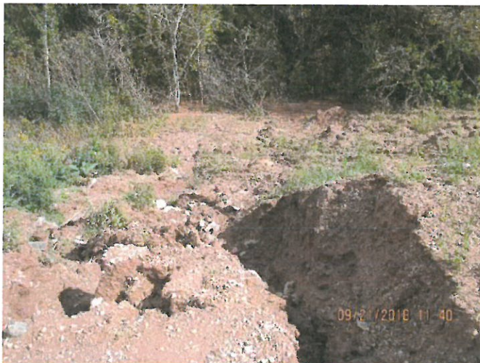
Photo 2: View of the north side of the disturbed area looking down into a wooded area where ponded turbid water is visible. Severe rill erosion is visible in the foreground. Photo direction is north and down.
