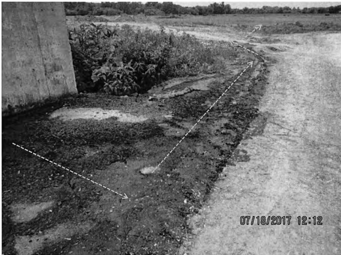
Photo 79: Alternate view of the north concrete wall of the feed storage area at the heifer site. Leachate was observed discharging from the wall and flowing west. Orange dashed arrows indicate flow path of leachate discharge. Photo direction is west.
