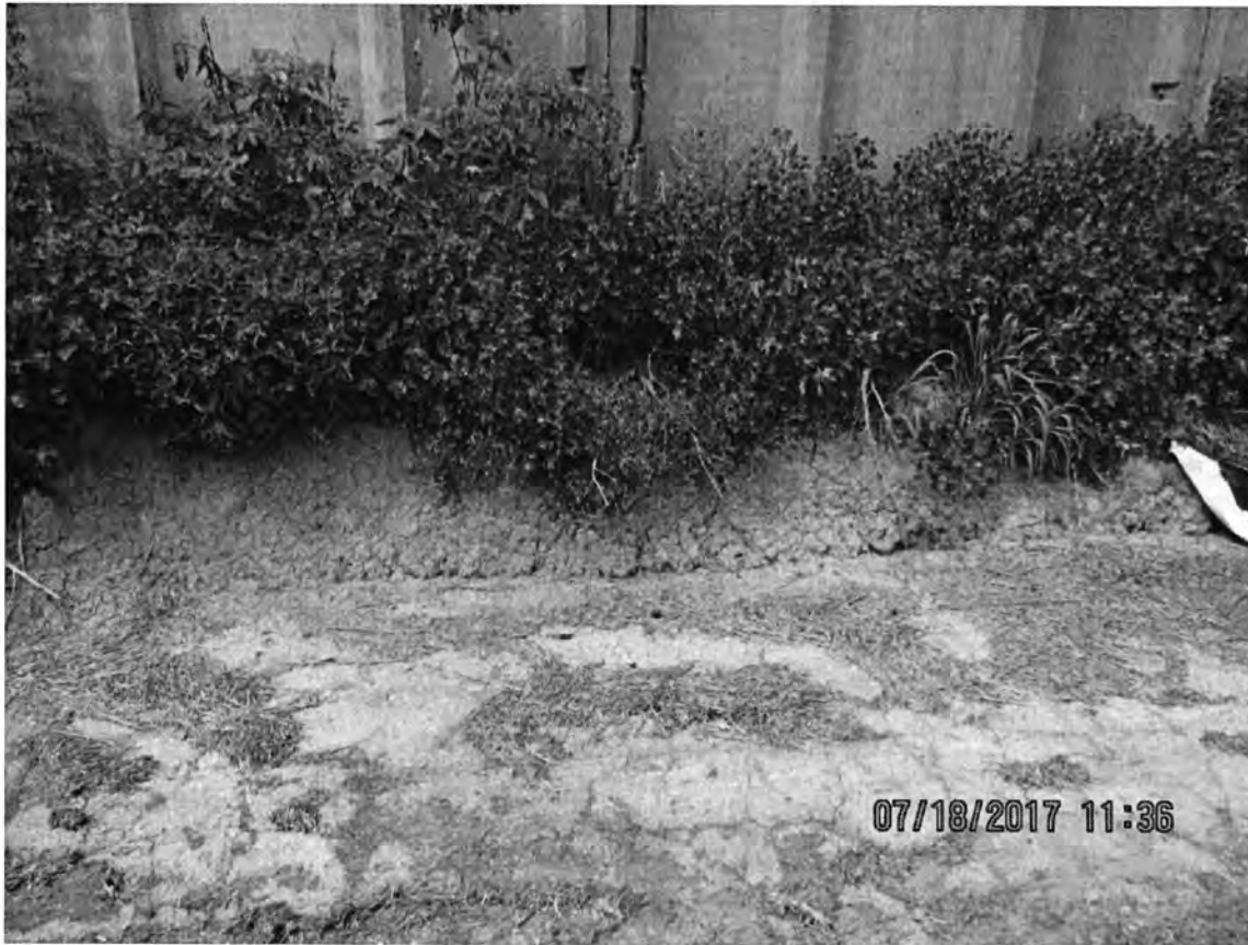
Photo 42: Close up view of the east wall of the feed storage area at the main farm site showing clay placed along the bottom of the wall to prevent leachate discharges. Photo direction is west and down.
