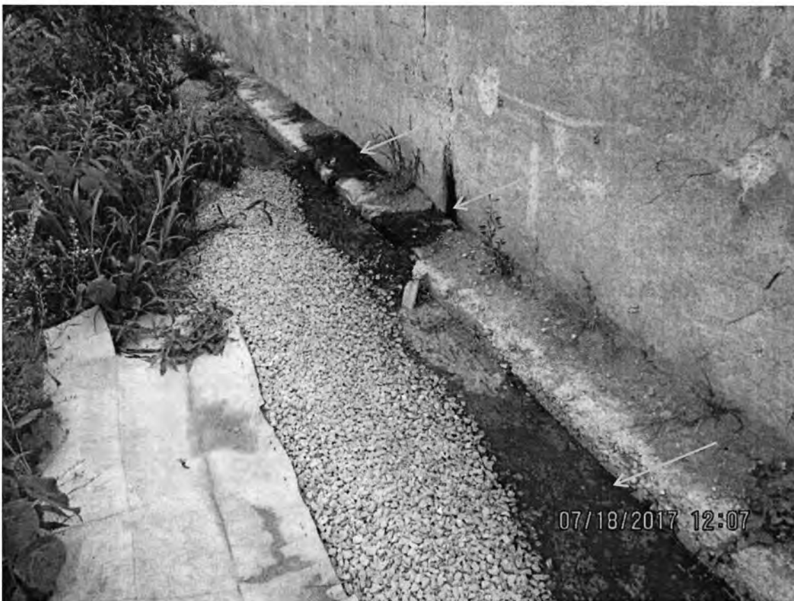
Photo 76: Close up view of the concrete wall on the NW side of the feed storage area at the heifer site. Leachate was observed discharging from the wall and was ponded adjacent to the wall (orange arrows). Photo direction is NE and down.
