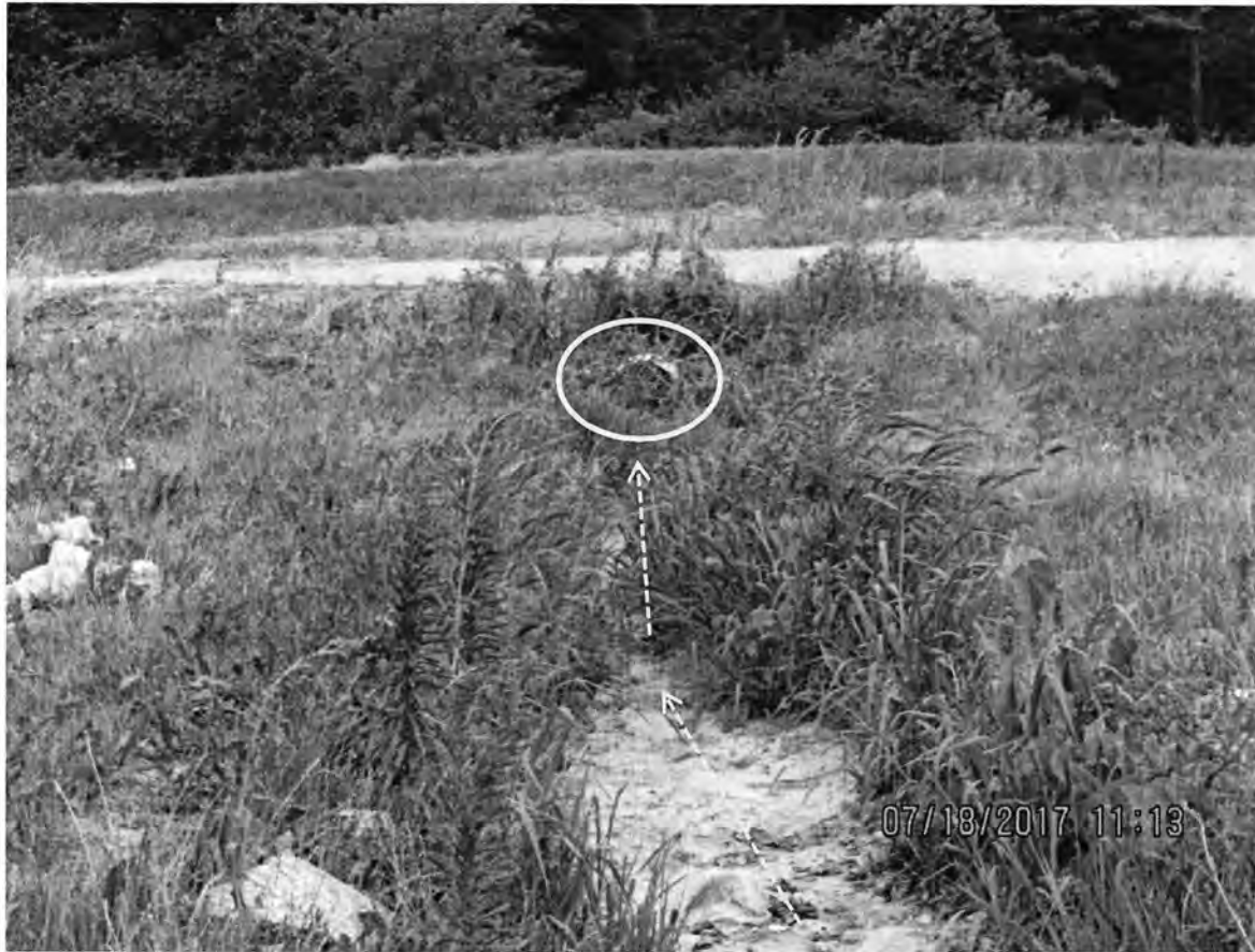
Photo 49: Close up view of the culvert through which storm water flows on the east side of the main farm in front of the freestall barn and milking parlor. Yellow dashed arrows indicate direction of flow path. Yellow circle is the culvert. Photo direction is north.
