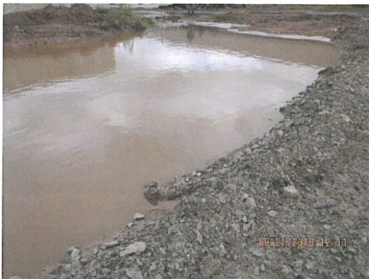
Photo 18: Close up view of the southern berm wall of the leachate/process wastewater collection basin south of the FSA. Photo direction is NE.
