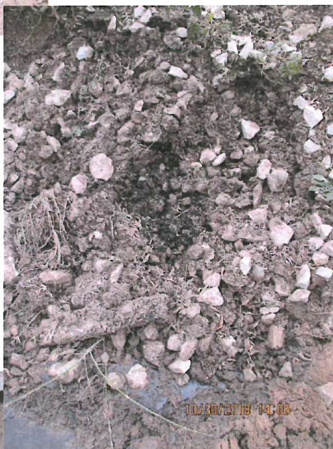
Photo 77 (right): Close up view of the stone, feed solids, and soil mixture piled against the exterior of the east wall of the FSA. Leachate seepage is visible. Photo direction is west and down.
