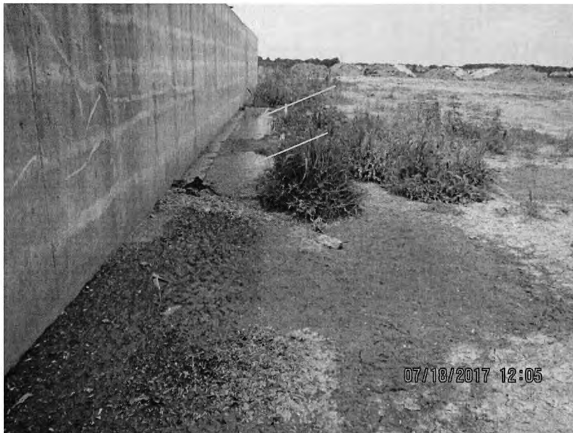
Photo 73: Close up view of a concrete wall from the middle of the feed storage area at the heifer site. Ponded leachate was observed adjacent to the wall (orange arrows). Photo direction is west.
