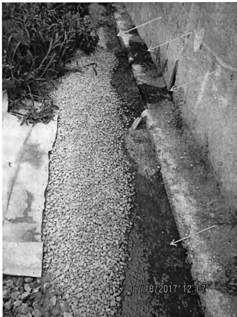
Photo 77: Alternate view of the concrete wall on the NW side of the feed storage area at the heifer site. Leachate was observed discharging from the wall and was ponded adjacent to the wall (orange arrows). Photo direction is NE and down.
