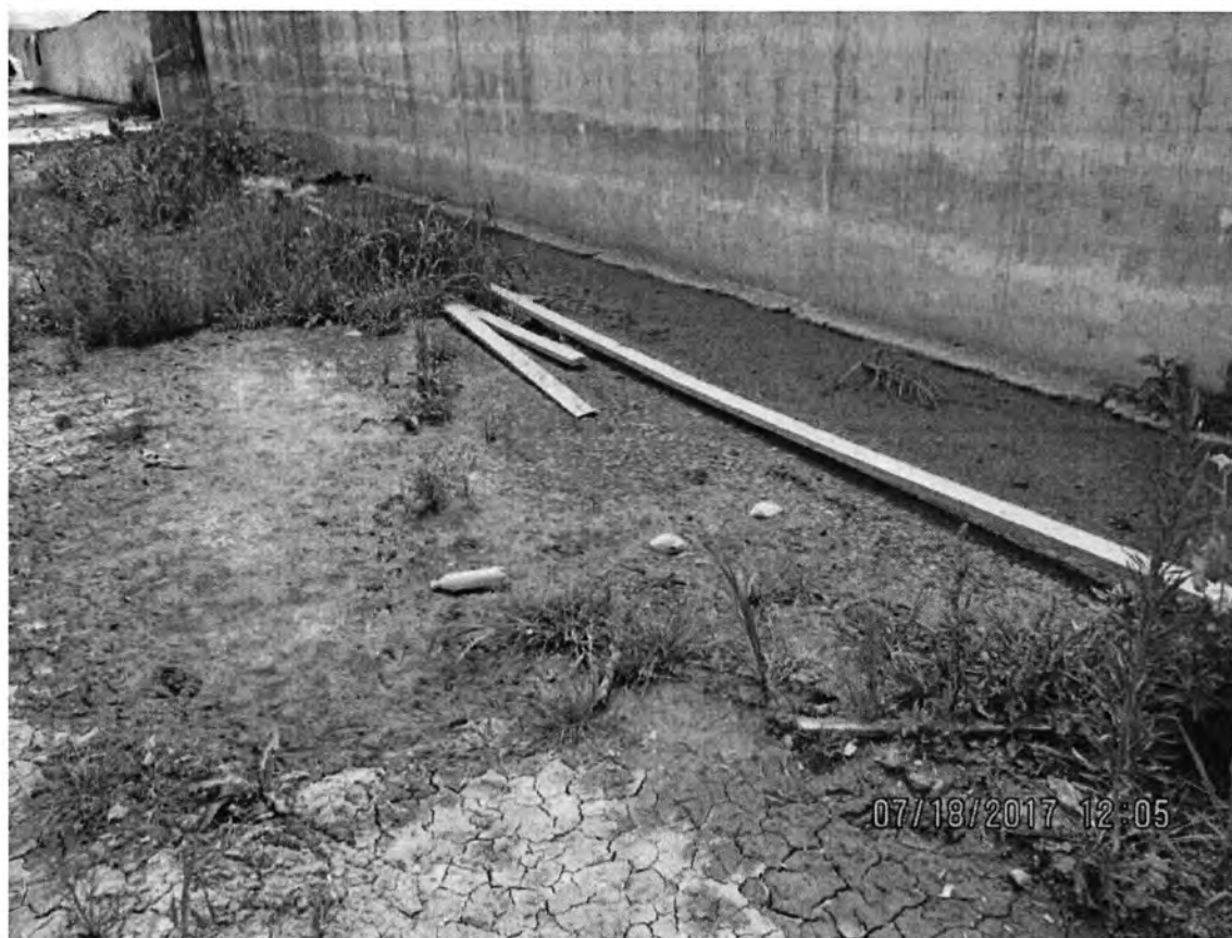
Photo 74: Close up view of a concrete wall from the middle of the feed storage area at the heifer site. Ponded leachate was observed adjacent to the wall. Photo direction is west.
