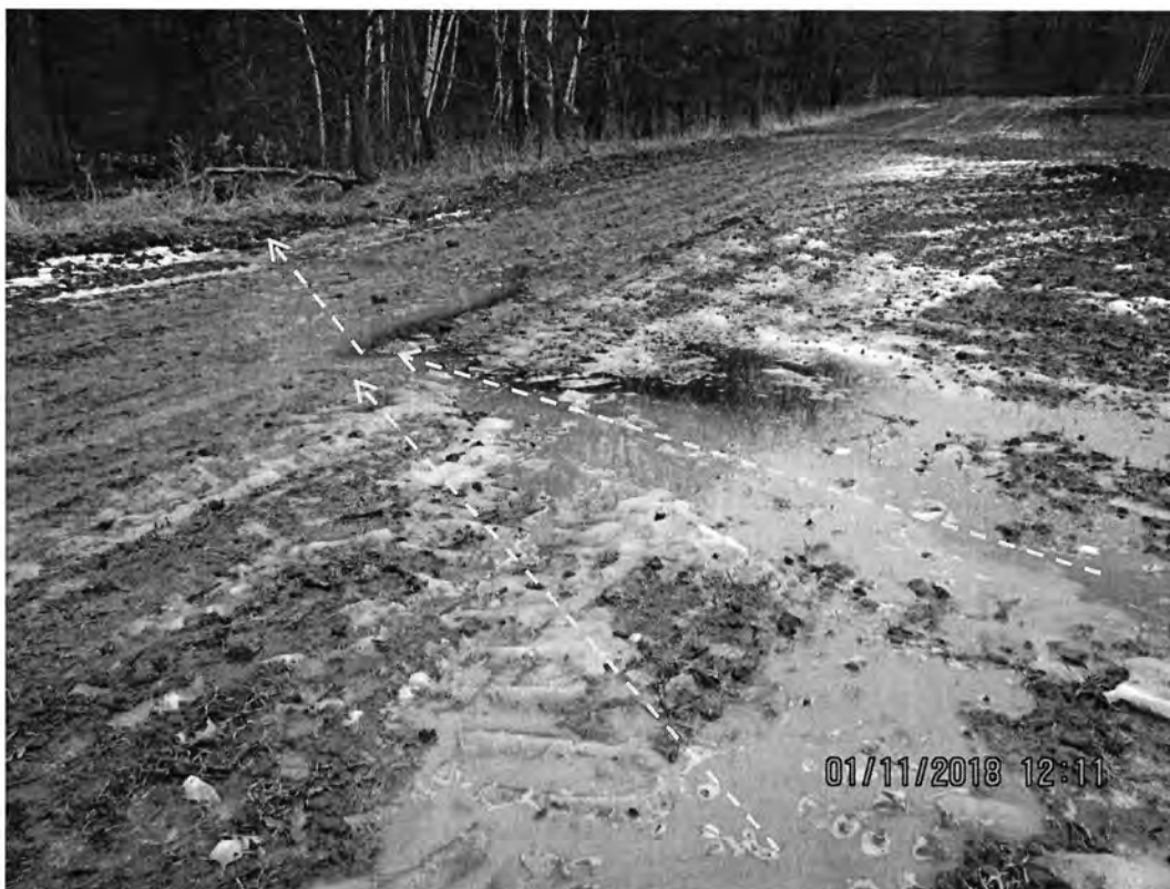
Photo 17: View of the northern section of 11J1&2 showing ponded storm water from snowmelt and the runoff flow path (indicated by the dashed yellow arrows). Photo direction is NE.
