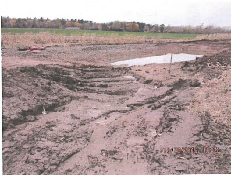
Photo 42: Closer view of the leachate/process wastewater collection basin south of the FSA, showing the regraded inlet area. Photo direction is SW.
