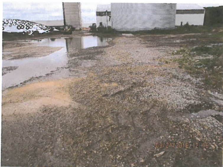
Photo 31: View of the gravel berm placed on the east side of the site between the steer barn and a grain bin to prevent discharges to the ditch at Lime Kiln Rd. Photo direction is north.
