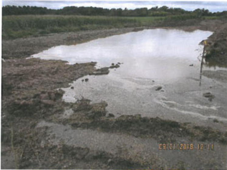
Photo 16: View of the leachate/process wastewater collection basin south of the FSA constructed to meet interim runoff control requirements. Photo direction is SW.
