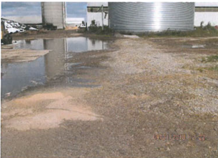
Photo 32: Alternate view of the gravel berm placed on the east side of the site between the steer barn and a grain bin to prevent discharges to the ditch at Lime Kiln Rd. Photo direction is north.
