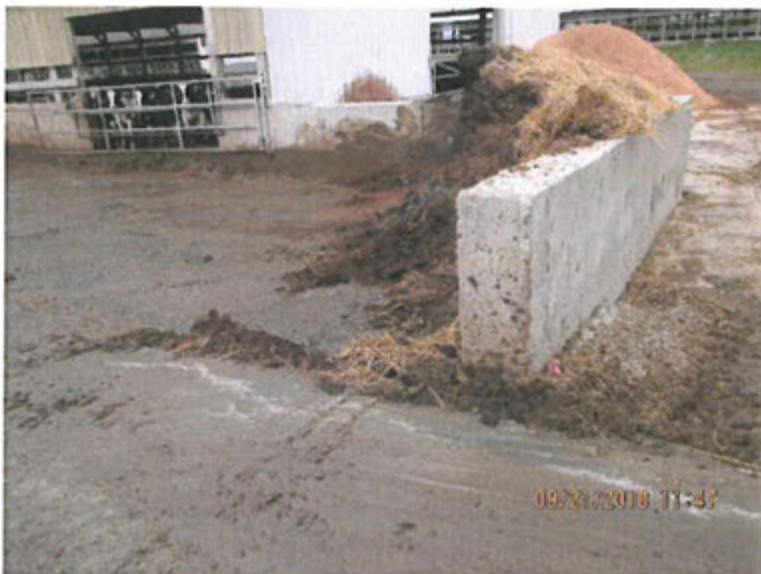
Photo 6: View of the east end of the concrete heifer lot where the northeast corner was enclosed with concrete walls as part of interim runoff control requirements. Photo direction is north/NW.
