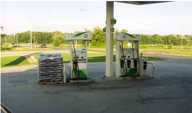
Non-compliant – Display is too high and too close to the dispenser
