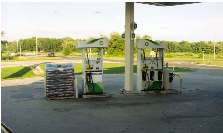
Non-compliant – Display is too high and too close to the dispenser
