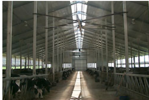
While High Volume Low Speed (HVLS) fans are normally recommended for loose housing applications, they may still be considered for modern and open free stall facilities. Photo: Midwest Rural Energy Council
