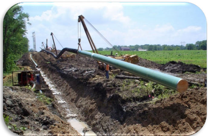
Figure 7: Lowering of pipe into open trench.
