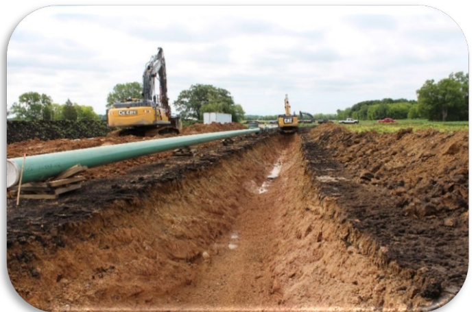
Figure 6: Open trench excavation.
