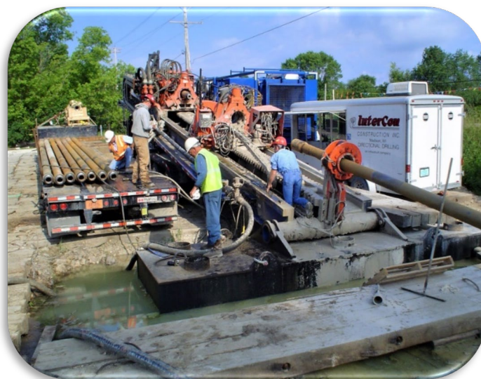
Figure 10: A horizontal directional drill machine.
