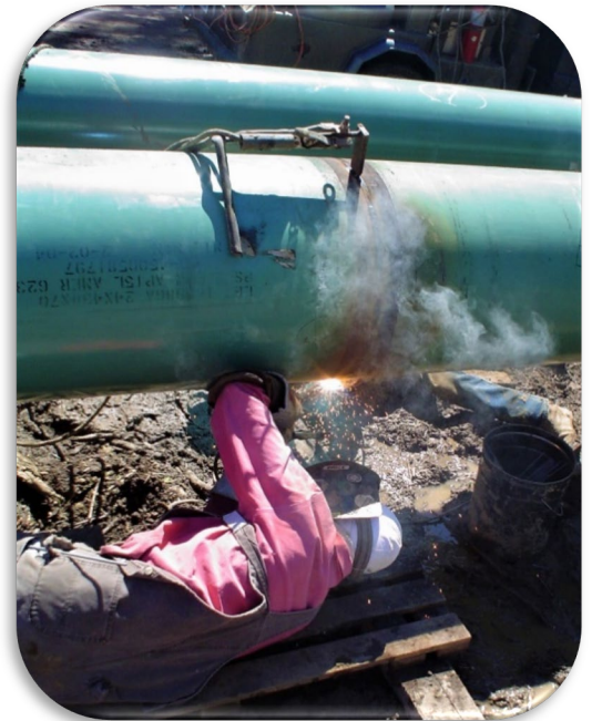
Figure 5: Pipe welding within the ROW.
