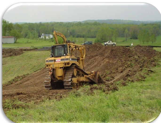
Figure 3: Topsoil stripping.
