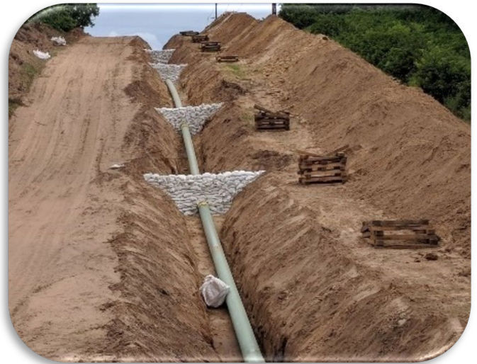
Figure 8: Placement of sandbag trench breakers.
