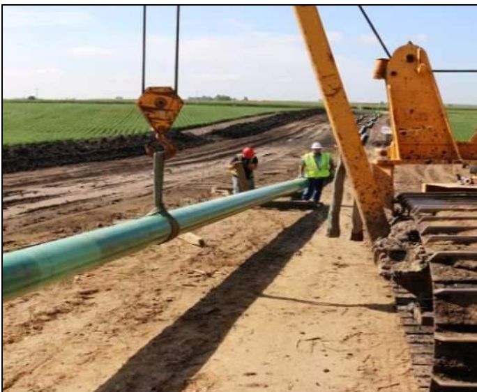
Figure 9: WPL Lowering-In Pipeline
