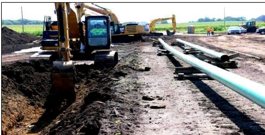
Figure 8: WPL Trench Excavation
