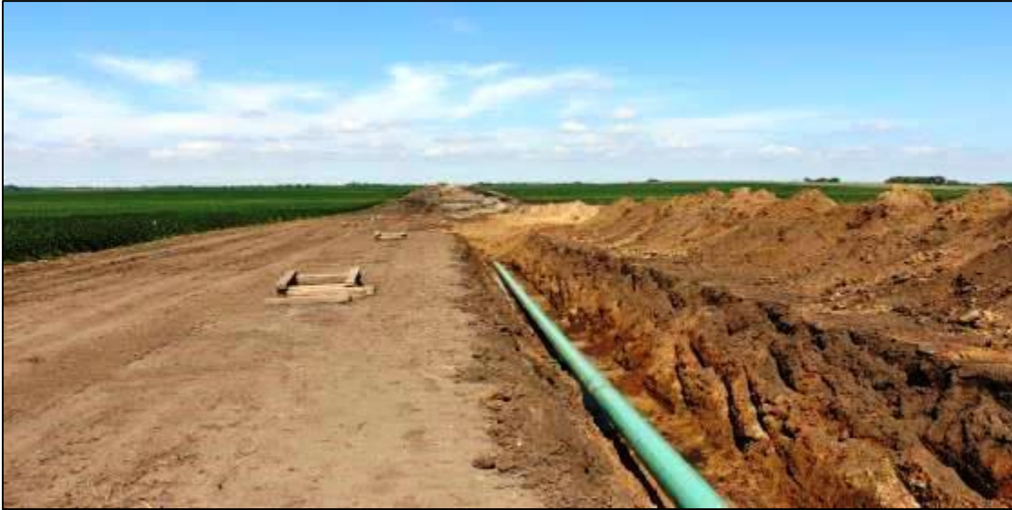
Figure 10: WPL Pipeline Installed in Trench
