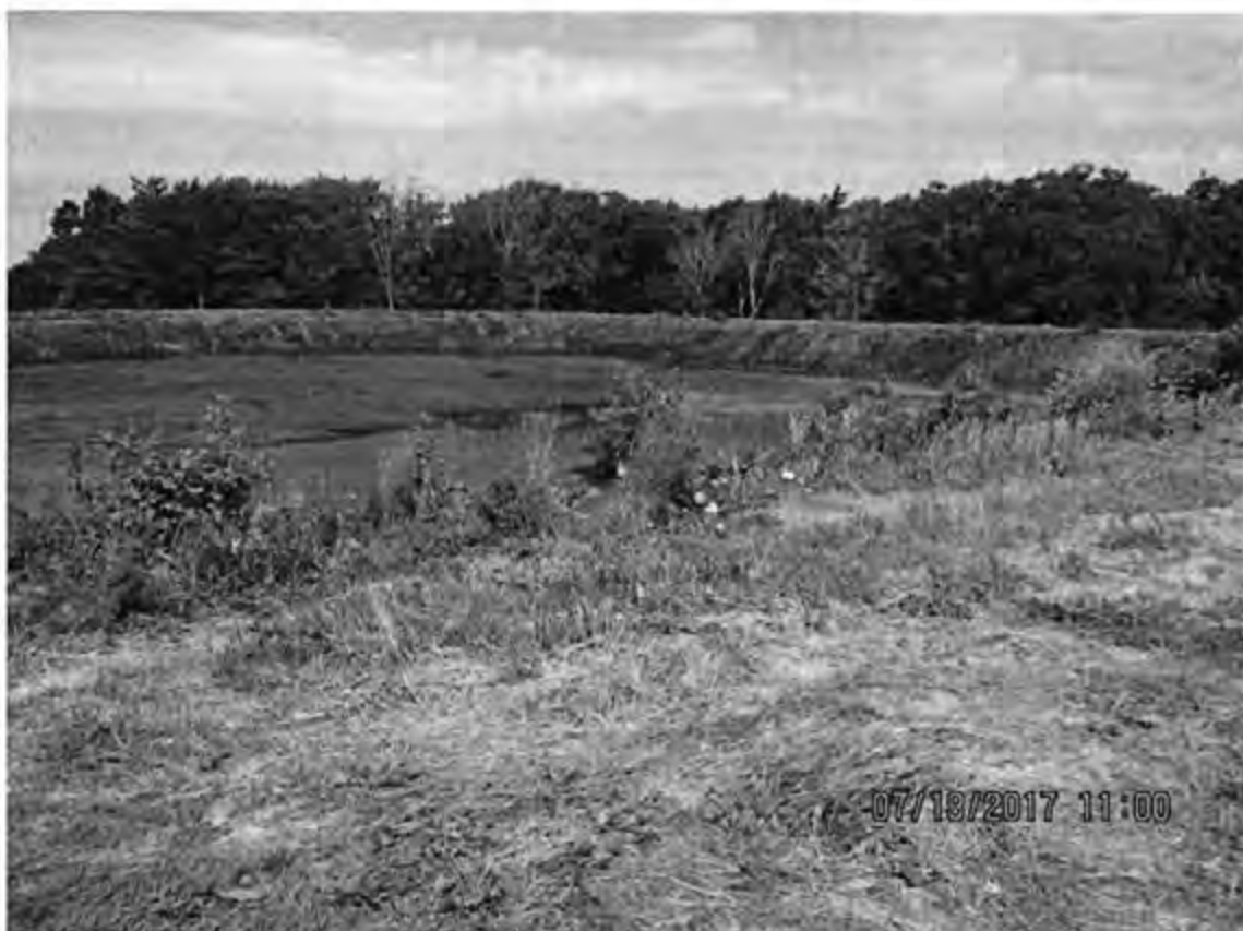
Photo 25: View of the middle and northern sections of outfall/WSF 001. Photo direction is NW.
