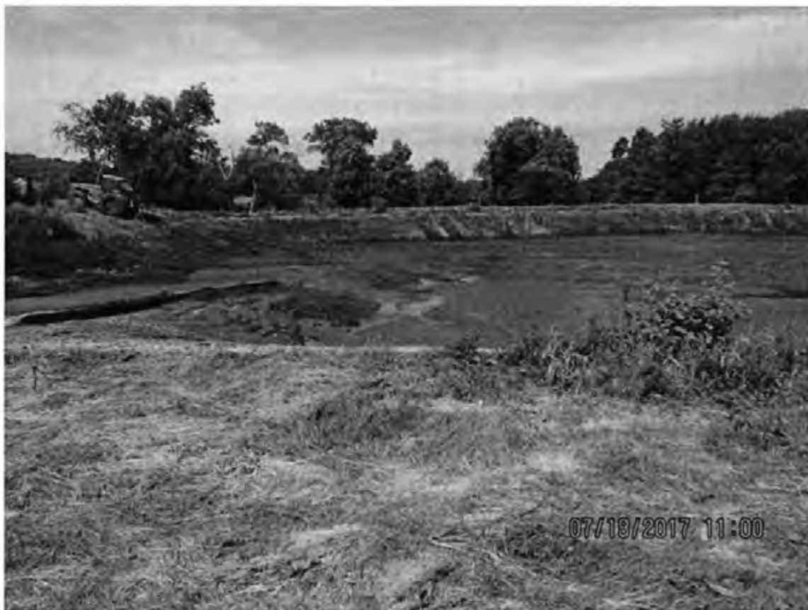
Photo 23: View of the southern and middle sections of outfall/WSF 001. Photo direction is west.
