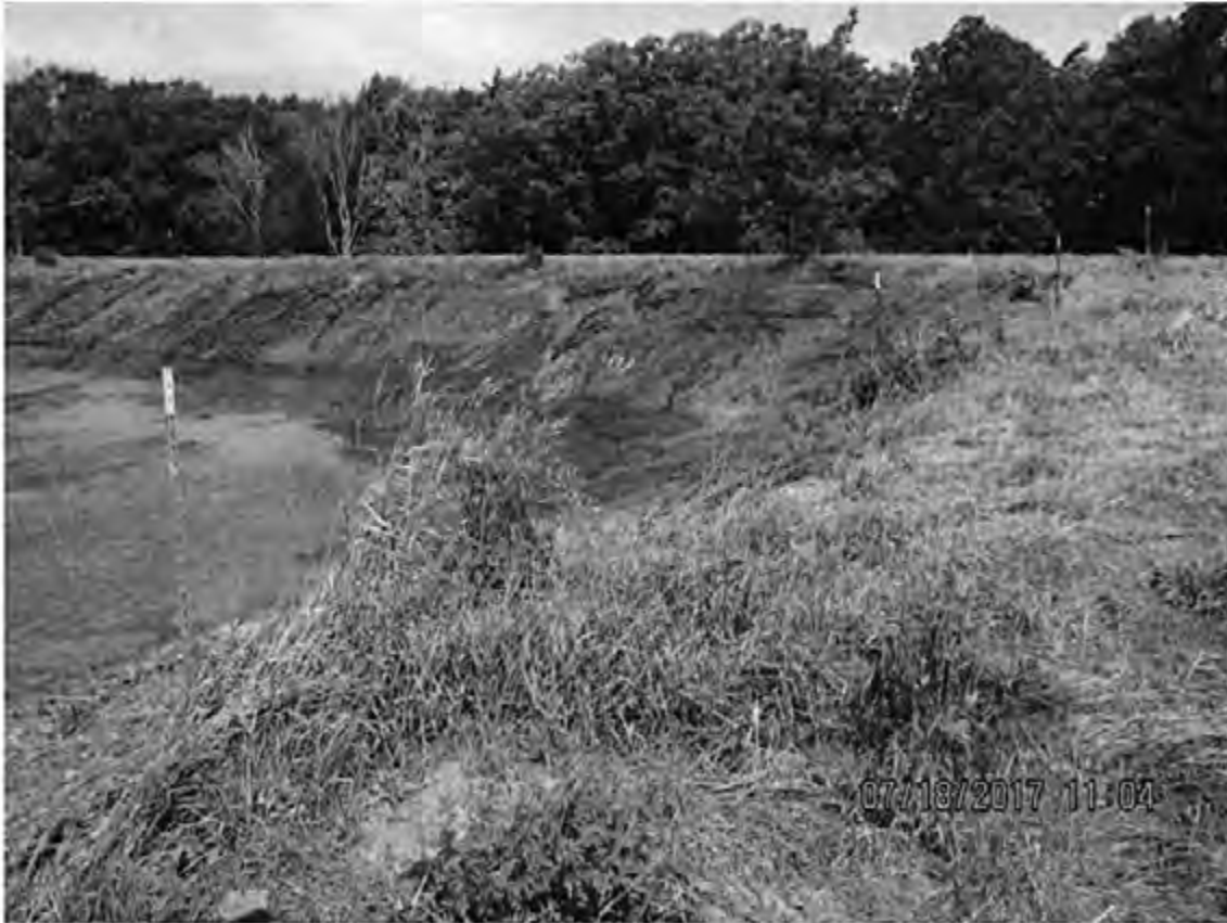
Photo 34: View of the NE corner of outfall/WSF 001. Photo direction is NW.
