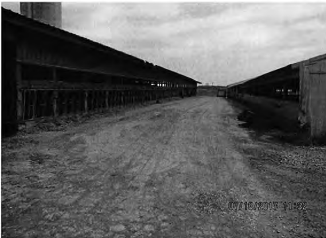
Photo 13: View of the concrete lane between the heifer/calf and maternity barns. Photo direction is east.
