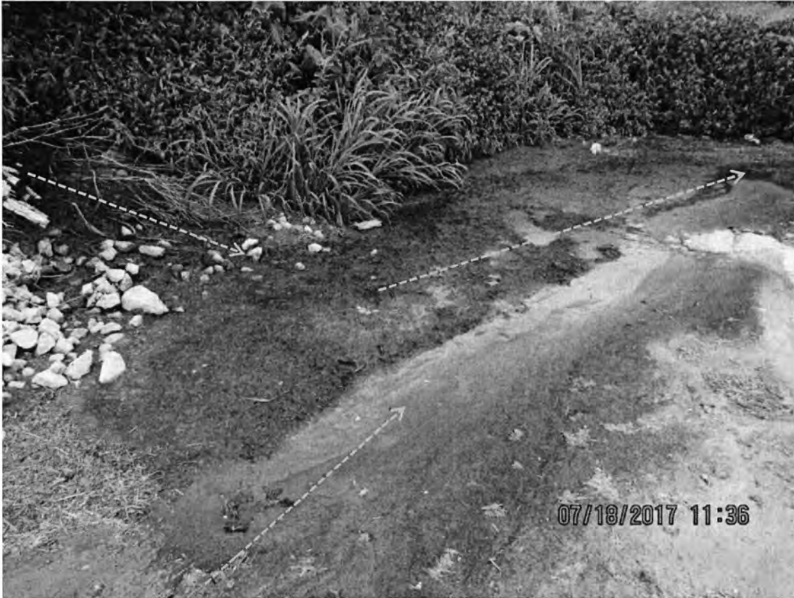
Photo 44: View of the leachate discharge from the NE corner of the feed storage area. Orange dashed arrows indicate the flow path and direction of leachate. Photo direction is north and down.
