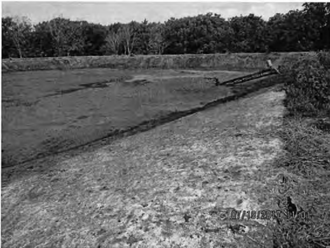
Photo 31: View of the northern section of outfall/WSF 001 showing the concrete ramp. Photo direction is NW.
