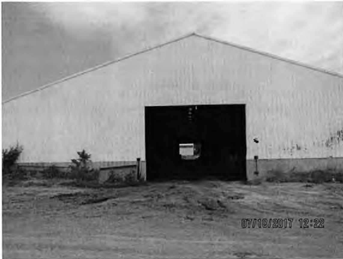
Photo 54: View of the south side of the large steer barn at the heifer site. Photo direction is north.
