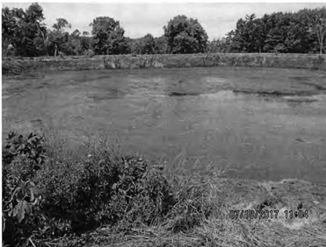
Photo 33: View of outfall/WSF 001. Photo direction is west.
