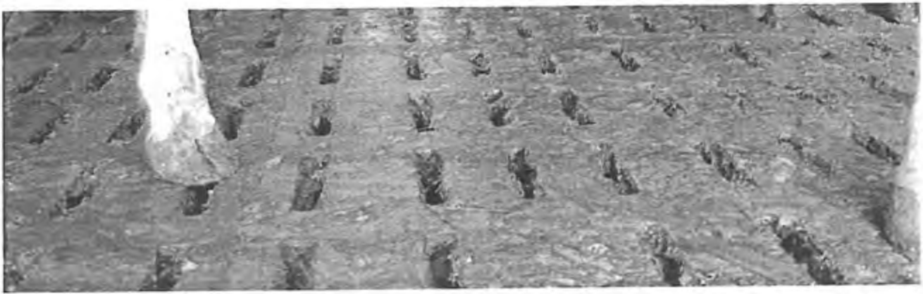
Figure 1. Slotted floors, like this example in a dairy barn, cover a manure storage that may be up to 10 feet deep, usually referred to as deep-pit storage.
