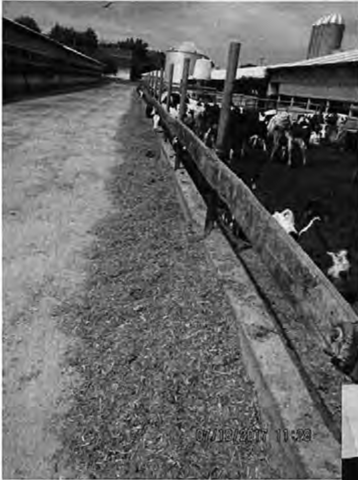
Photo 15: View of the heifer/calf barn feedlot. Photo direction is west.
