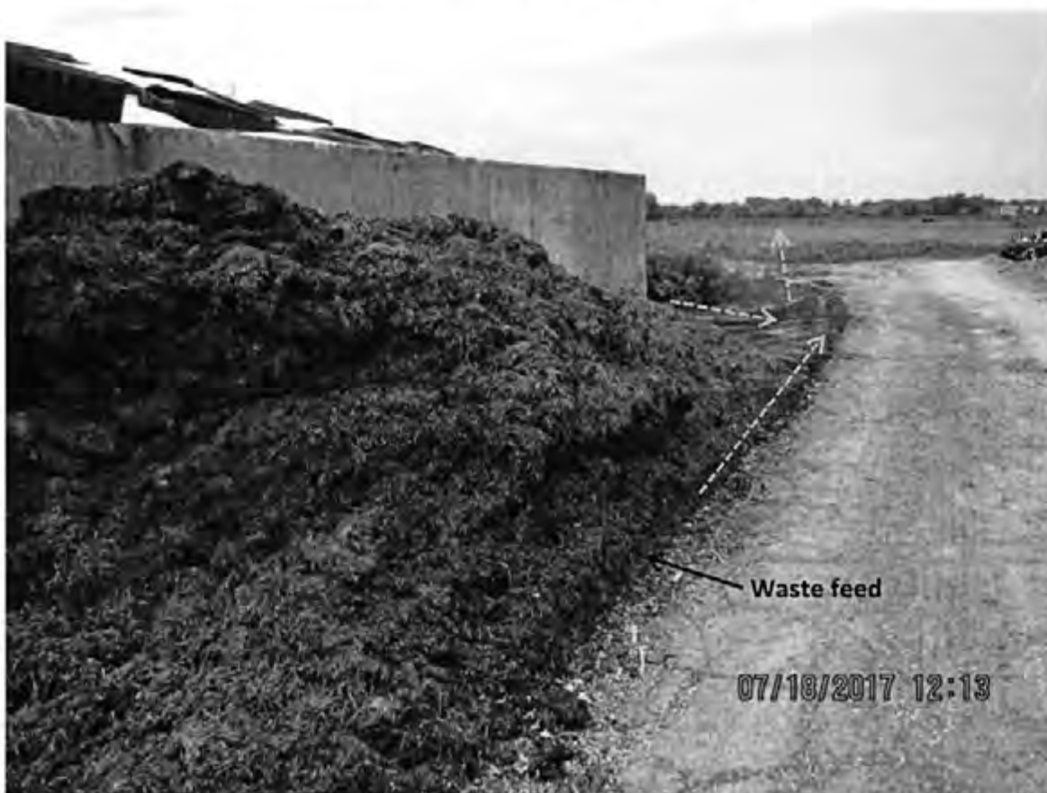
Photo 80: Alternate view of the north concrete wall of the feed storage area at the heifer site. Leachate was observed discharging from the wall and flowing west. Orange dashed arrows indicate flow path of leachate discharge. Photo direction is west.
