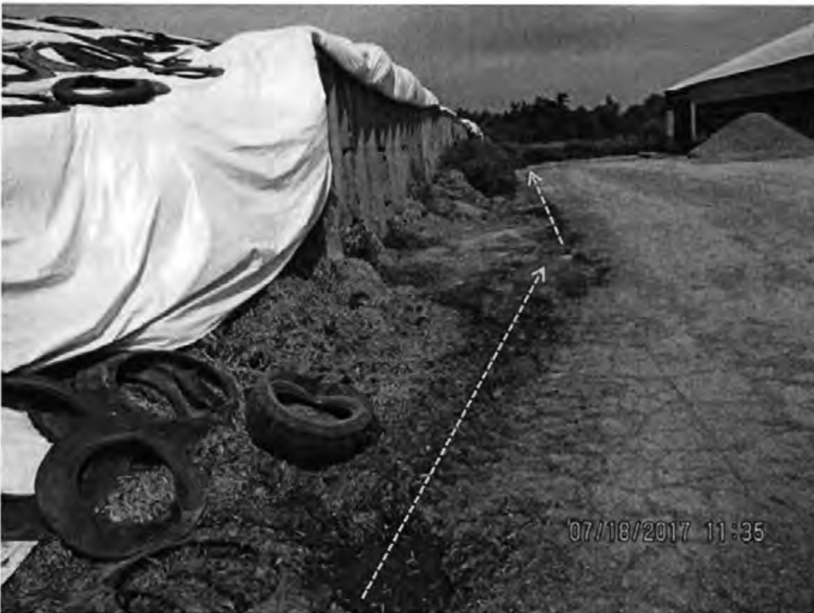
Photo 41: View of the east wall of the feed storage area at the main farm site. Leachate is visible discharging from the feed storage area. Orange dashed arrows indicate the flow path and direction of leachate. Photo direction is north.
