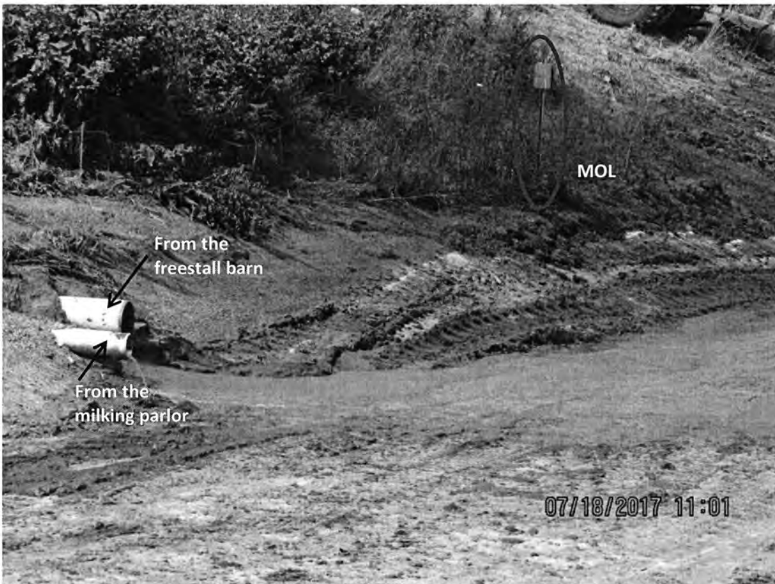
Photo 27: Close up view of the MOL and manure transfer system discharge pipes in the southern section of outfall/WSF 001. Photo direction is west and down.
