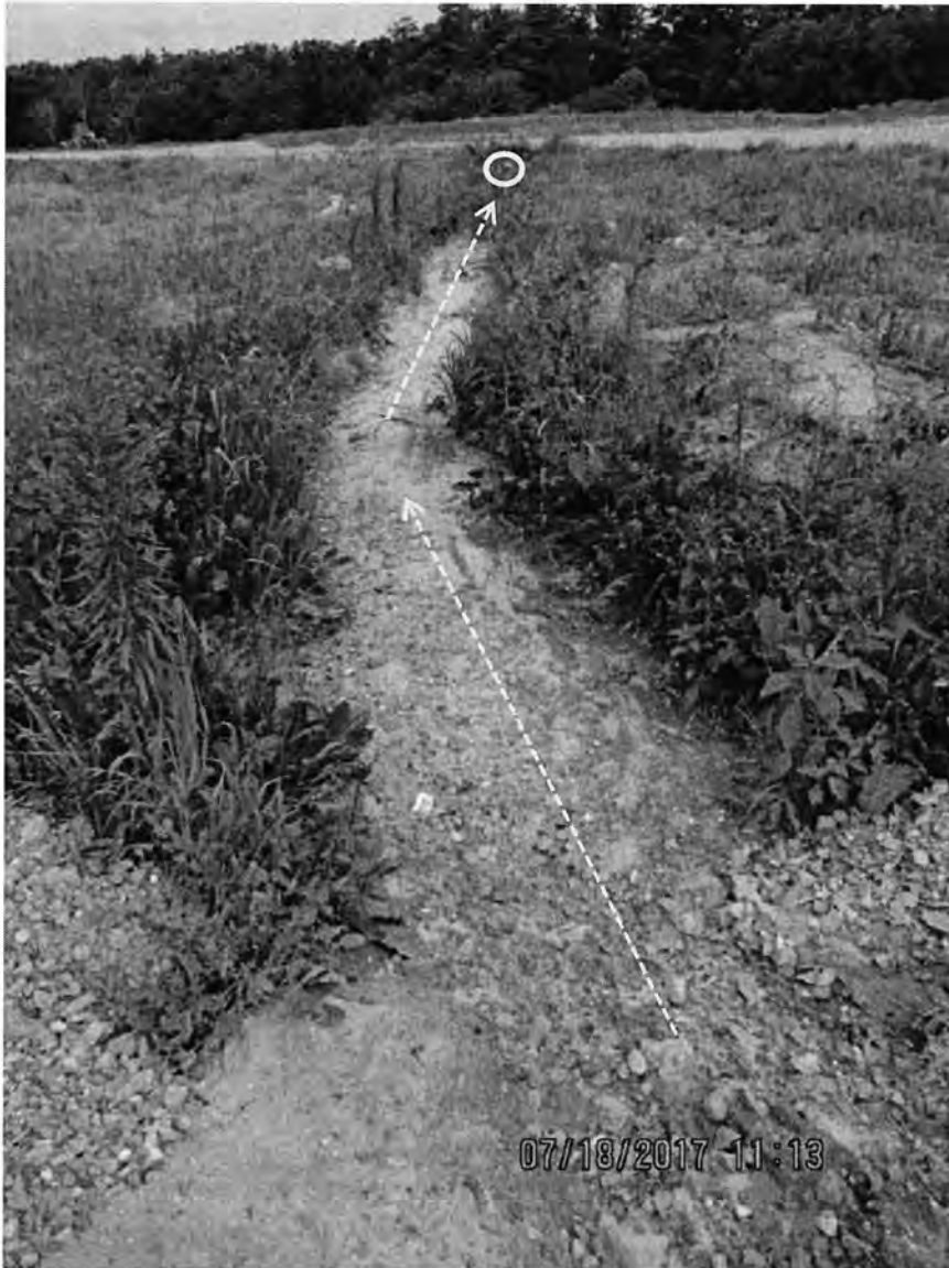
Photo 48: View of the storm water flow path on the east side of the main farm in front of the freestall barn and milking parlor. Yellow dashed arrows indicate direction of flow path. Yellow circle is a culvert. Photo direction is north.
