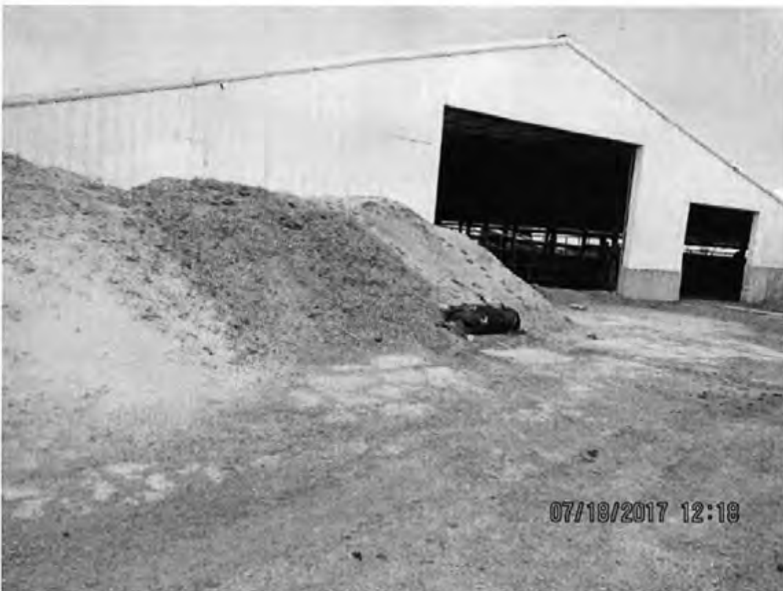
Photo 51: View of the east side of the heifer barn at the heifer site. Bedding pile and animal mortality are visible. Photo direction is NW.
