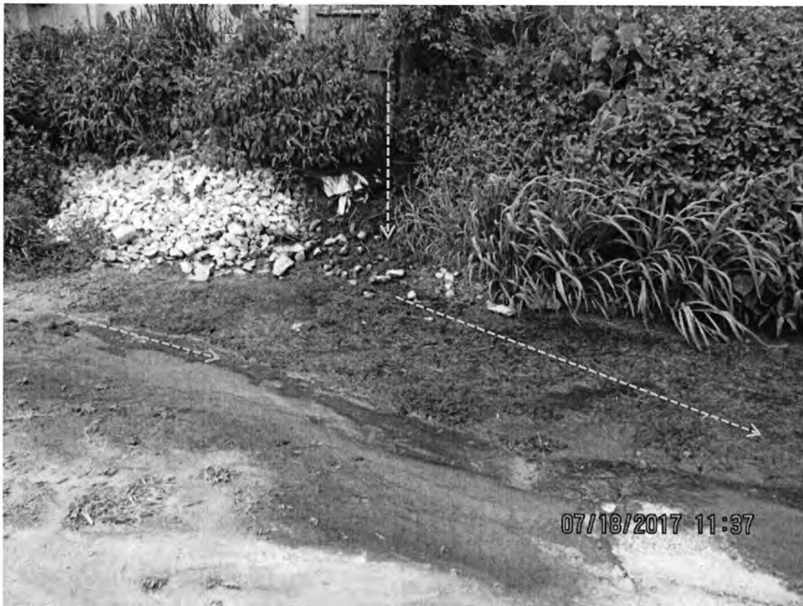
Photo 43: View of the leachate discharge from the NE corner of the feed storage area. Orange dashed arrows indicate the flow path and direction of leachate. Photo direction is SW and down.
