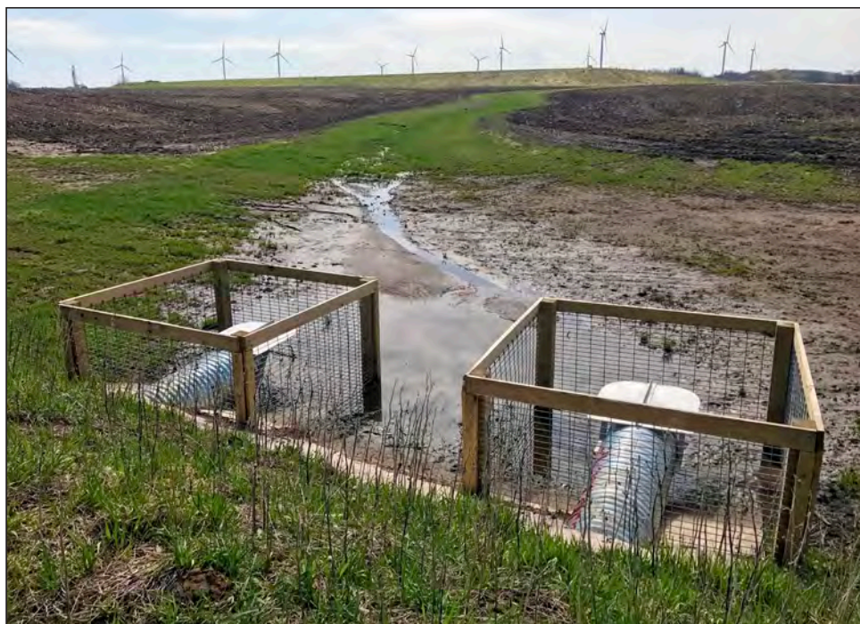
Hooded inlet pipes, looking upstream to the grassed waterway
